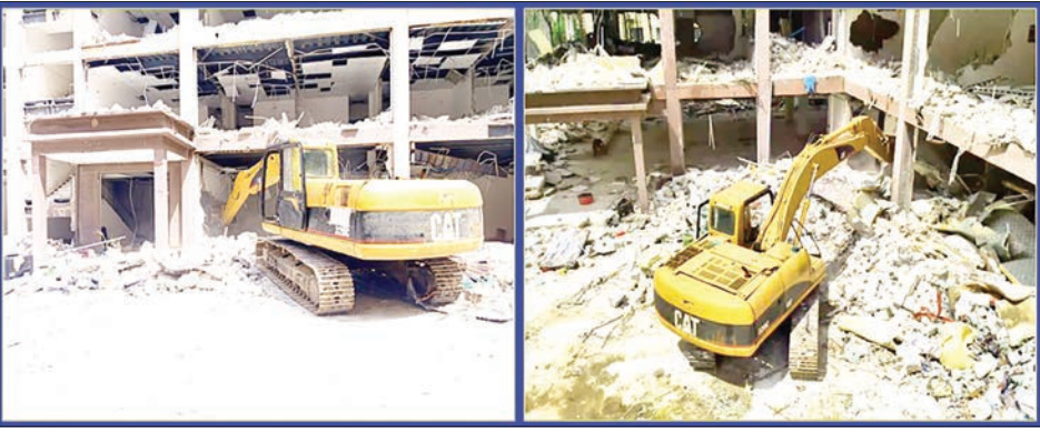
Images reveal systematic demolition of a five-storey scam-related building in the Shwe Kokko Phase II crackdown.
