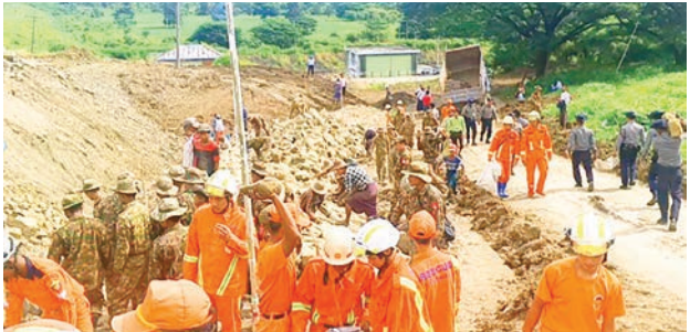
The Ma Mya Dam in Myanaung, Ayeyawady Region.
