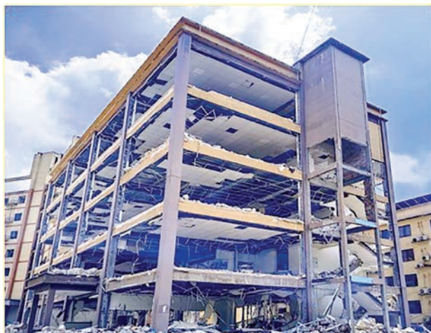
New image reveals the ongoing demolition of scam-related structures, buildings, and facilities in the Shwe Kokko area, Myawady, Kayin State.
